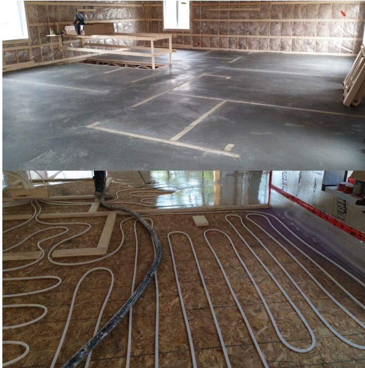
When installing tubing in less than 2½ inches of concrete, we recommend first installing the bottom plates for your interior walls before laying the pipes. Take care not to lay tubing less than 6 inches from an exterior or interior wall, to prevent damage during construction. Although these measures are less essential when installing tubing in a thicker slab, you should still remain vigilant when working near heating pipes.
