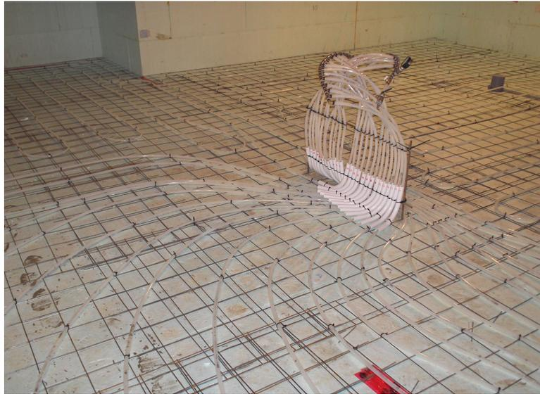
Before pouring the concrete, you should always check for leaks in the PEX tubing. It may have been damaged during installation.
