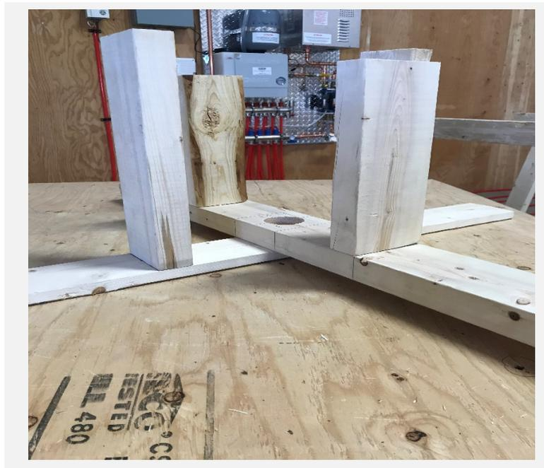
8- Then, arrange the remaining one-by-four and two-by-four in the shape of a cross. Be sure the holes at the centre of the two boards line up. Set this piece aside.
